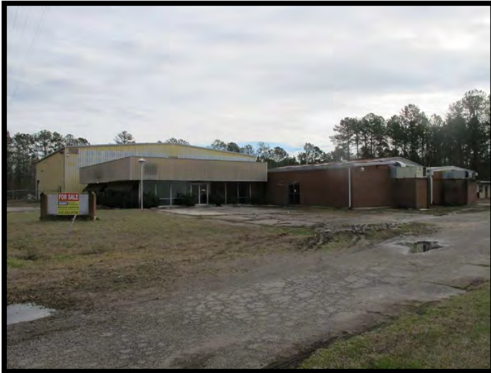
NS1543 – View of Commercial Building, 105 Gelo Road, Looking Southeast.
