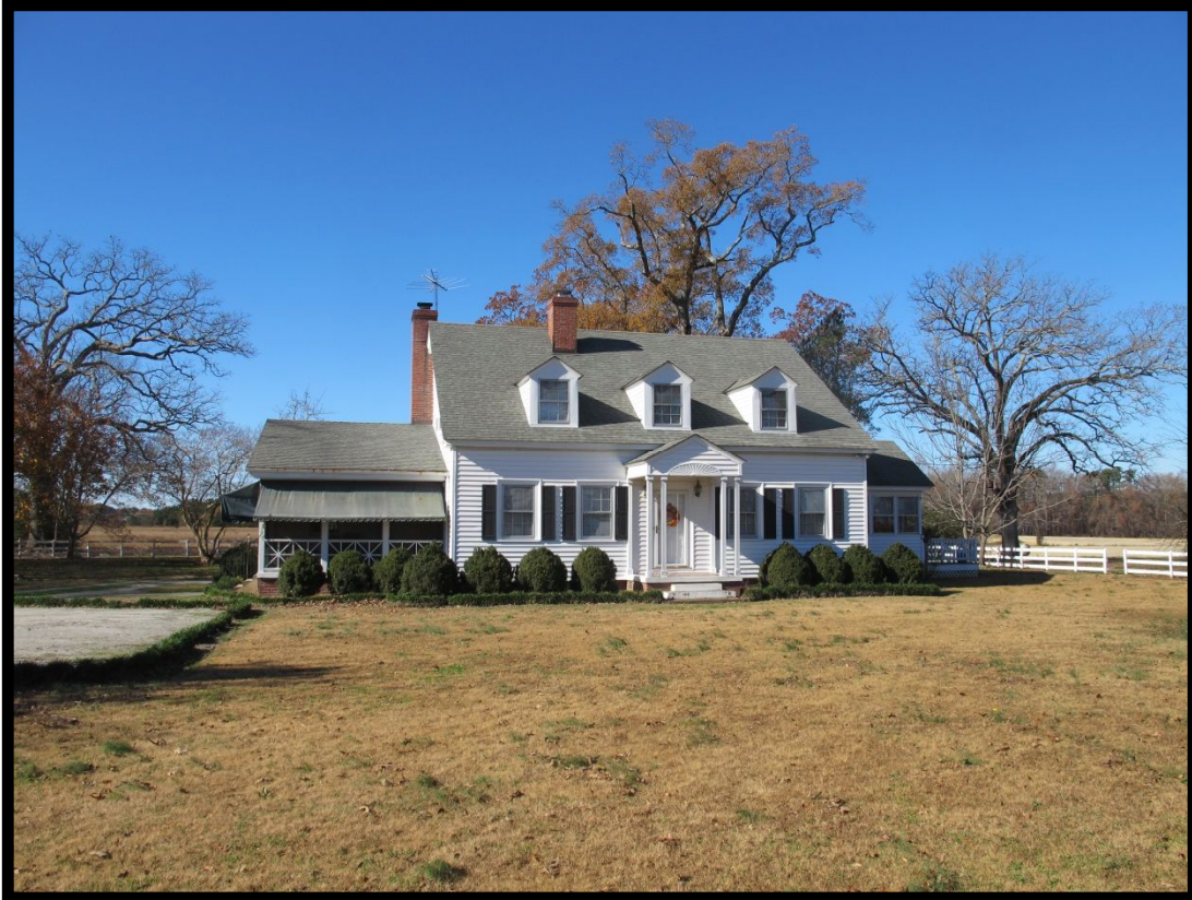
Figure 4.4 William W. Flye House (A), Looking Northwest
