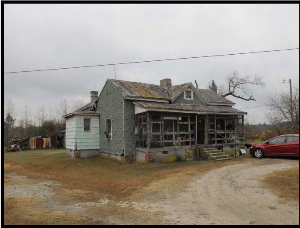
ED1646 – View of Jones Tenant House, Looking Northwest
