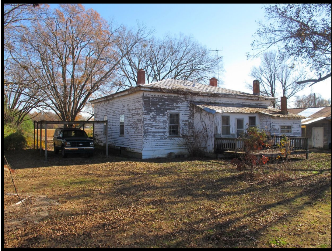
Figure 4.8 Henry E. Odom House (B), Looking Southeast
