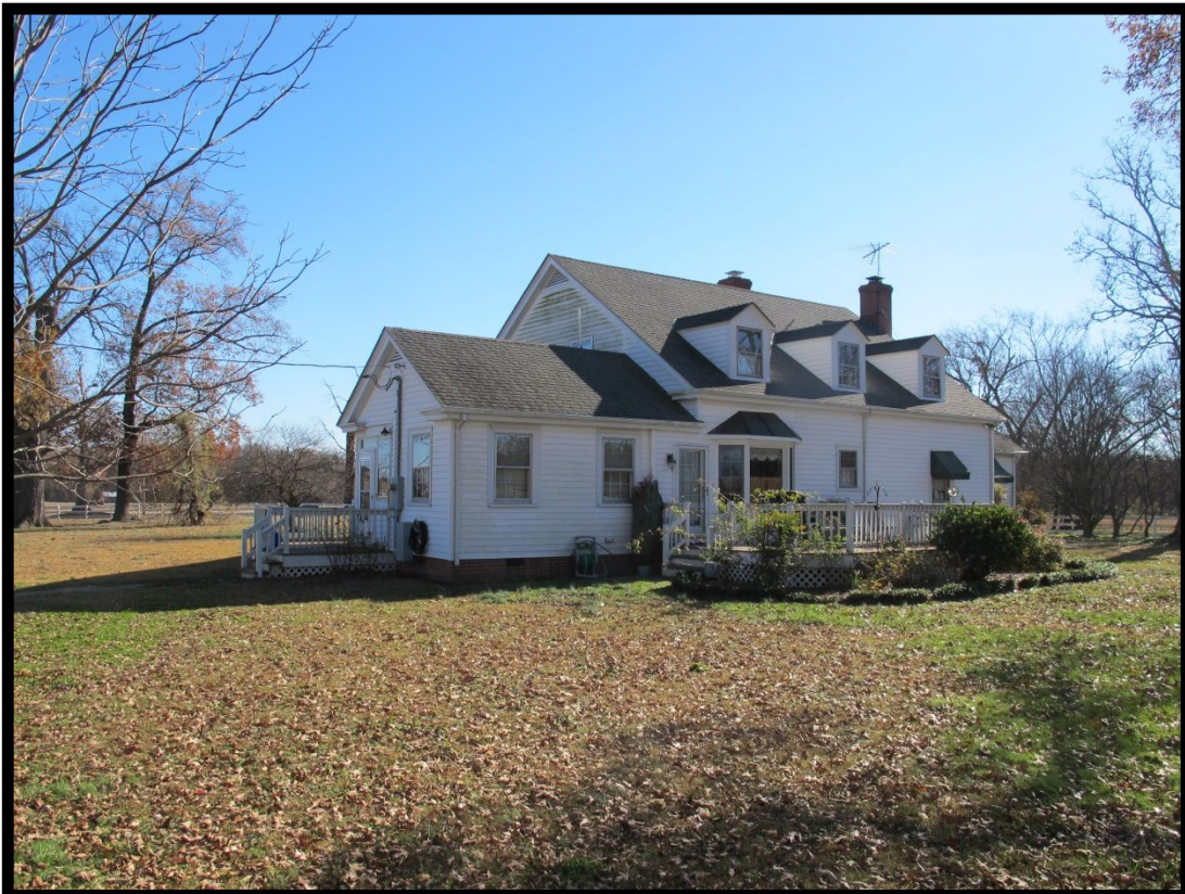
Figure 4.5 William W. Flye House (A), Looking Southeast
