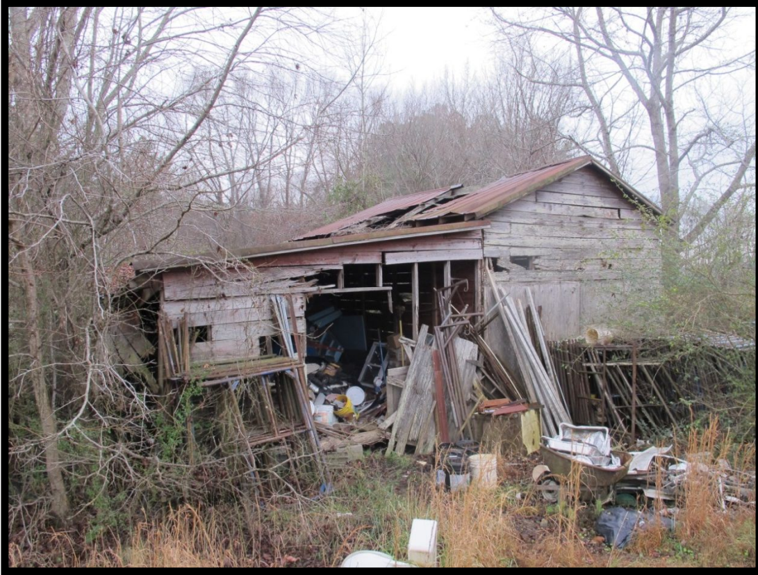
Figure 4.69 Jones Tenant House, View of Outbuilding, Looking Southwest
