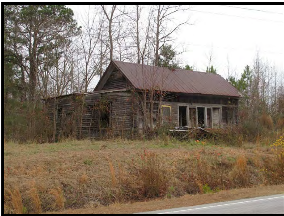
NS1534 – View of House, N. Wesleyan Blvd (US 301), Looking Northwest.
