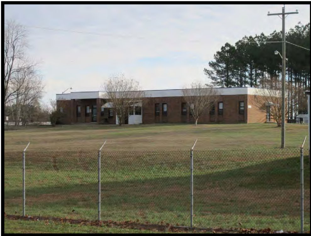
ED0623 – View of Administrative Building Associated with the School (built before 1974), Looking Northeast.
