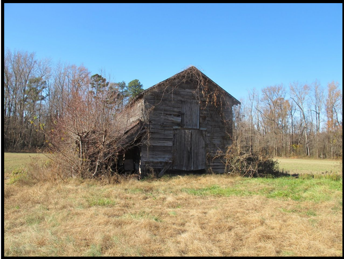
Figure 4.50 Outbuilding Associated with Tenant House (Q), Looking Northwest
