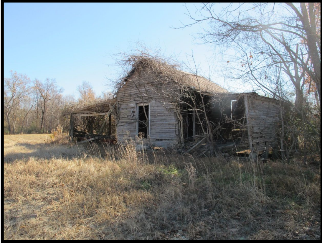
Figure 4.30 Outbuilding Associated with Tenant House (H), Looking Southeast
