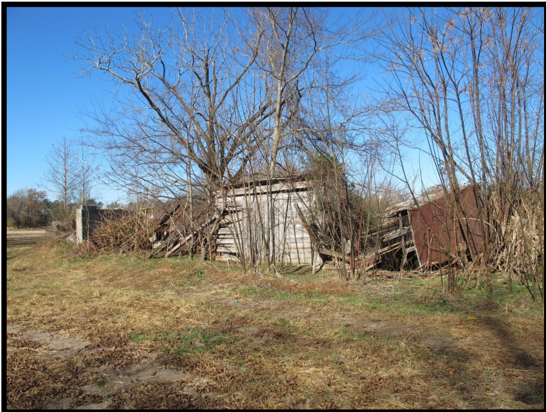
Figure 4.23 Outbuilding at Henry Odom Tenant House, Looking Northwest
