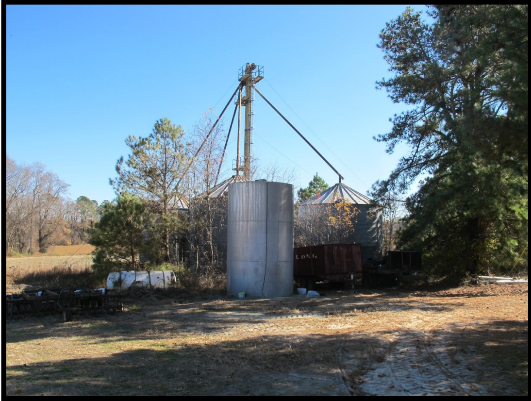
Figure 4.46 Silos East of Tenant House (O), Looking Southeast
