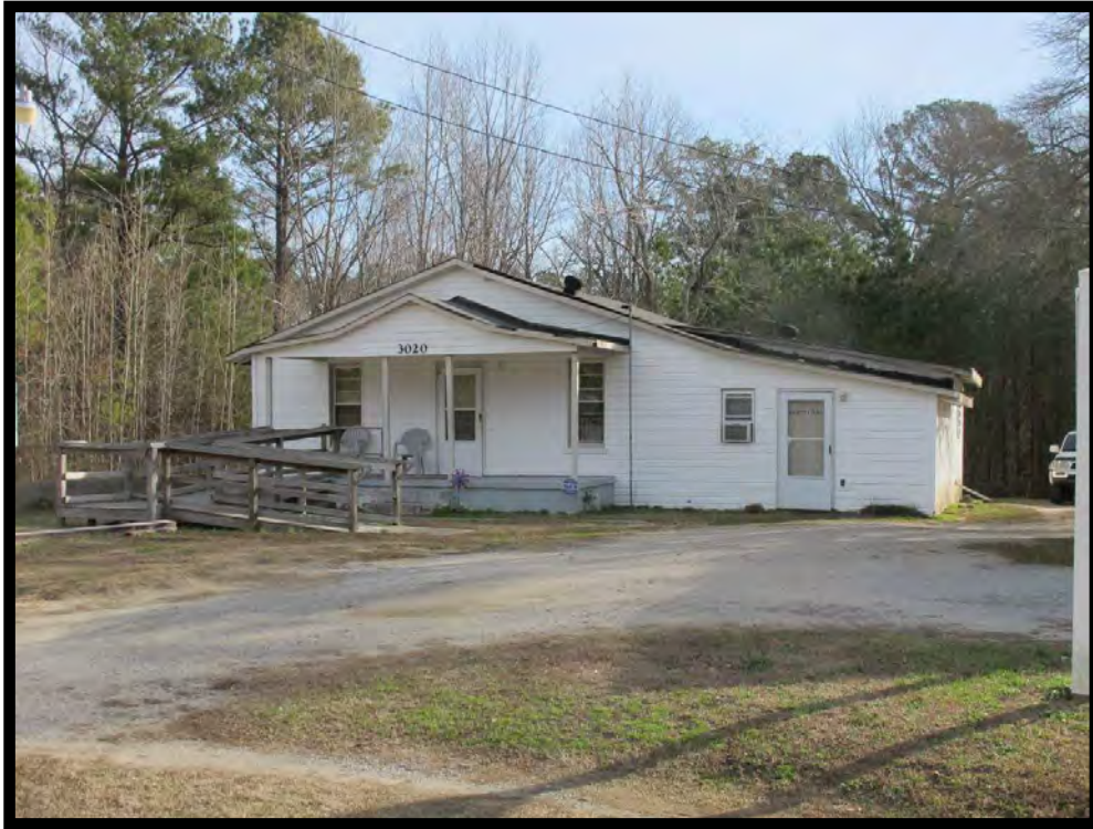
NS1537 – View of House & Store, 3020 N. Wesleyan Blvd (US 301), Looking Northeast.
