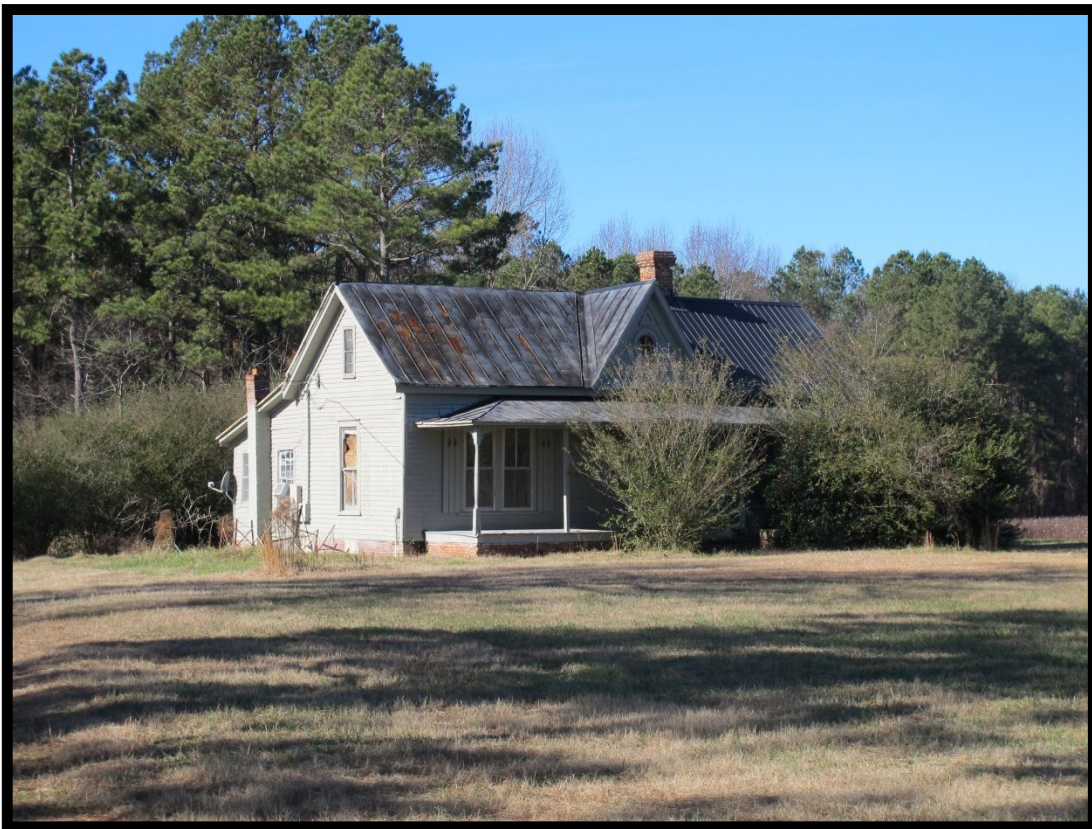
Figure 4.77 House at 10098 NC 48, Nash County, Looking Northwest (Not in APE)
