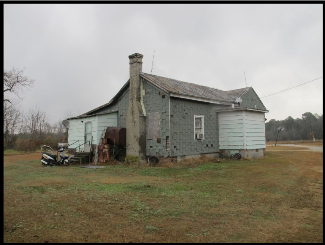
Figure 4.62 Jones Tenant House, Looking Northeast.
