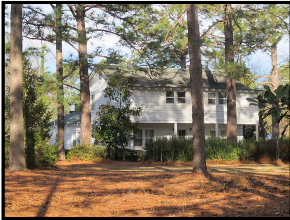
ED1641 – View of House, 4232 Old Battleboro Road, Looking Northwest.
