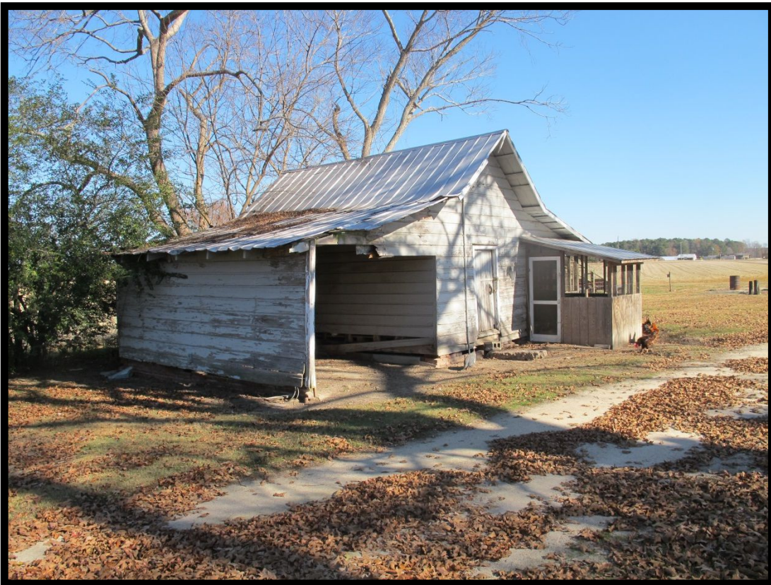
Figure 4.9 Outbuilding (aa), Looking Northeast
