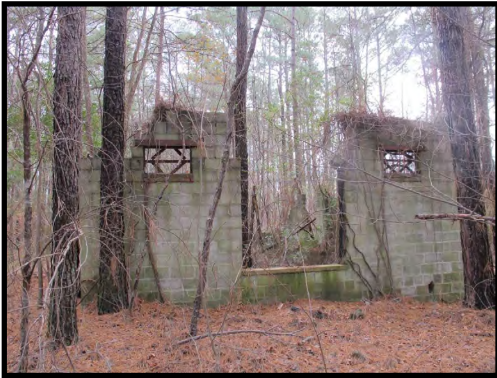
ED1651 – View of Commercial Building, 12601 NC 97 West, Looking East.
