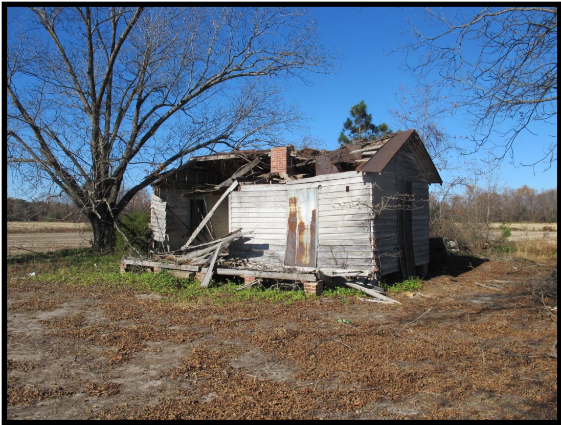
Figure 4.26 Tenant House (G), Looking Northwest
