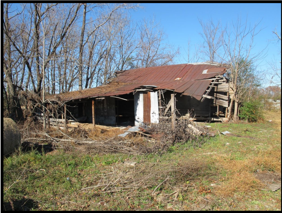
Figure 4.24 Pack House at Henry Odom Tenant House, Looking Northwest
