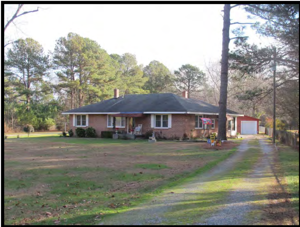
ED1643 – View of House, 4005 Old Battleboro Road, Looking Northeast.
