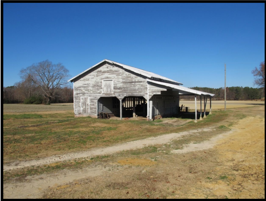
Figure 4.10 Outbuilding (bb), Looking Northwest
