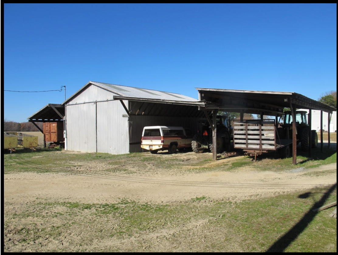
Figure 4.37 Machine Shed (K), Looking Northwest (Outside Project Area, Within APE)
