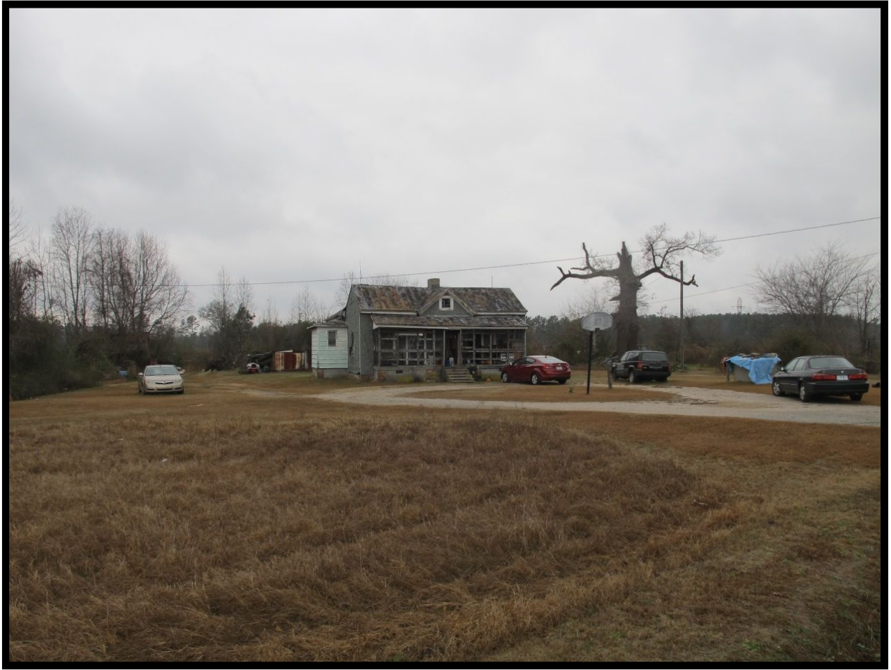
Figure 4.59 Jones Tenant House, Looking Northeast
