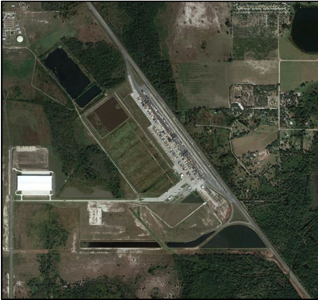
Figure 1.2 View of Existing CSX Intermodal Facility in Winter Haven, Florida
