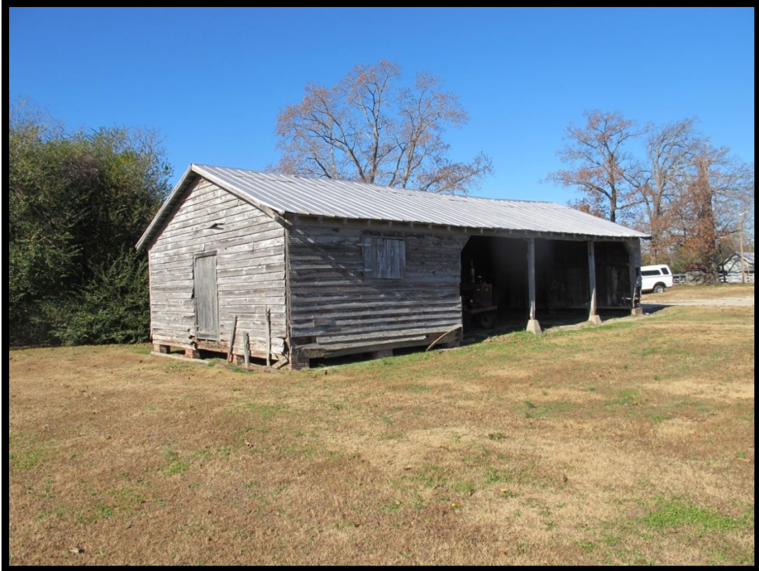
Figure 4.12 Machine Shed (dd), Looking Northwest
