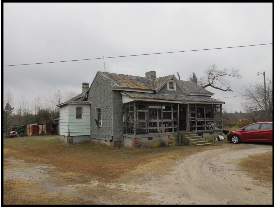
Figure 4.61 Jones Tenant House, Looking Northwest.
