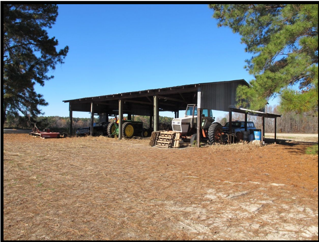
Figure 4.45 Machine Shed East of Tenant House (O), Looking Northwest (Outside Project Area, Within APE)
