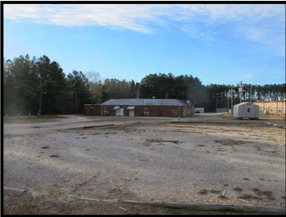
ED0623 – View of Utility Building Associated with the School, Looking Southeast.
