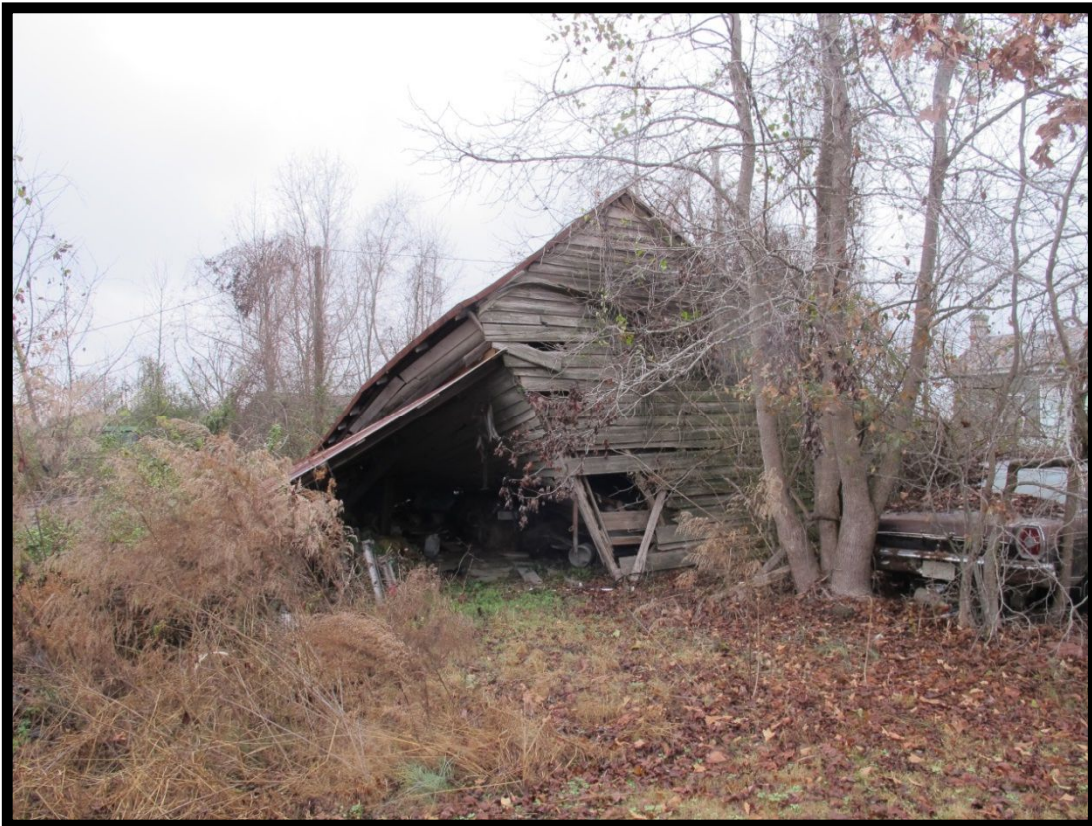
Figure 4.68 Jones Tenant House, View of Outbuilding, Looking Northwest
