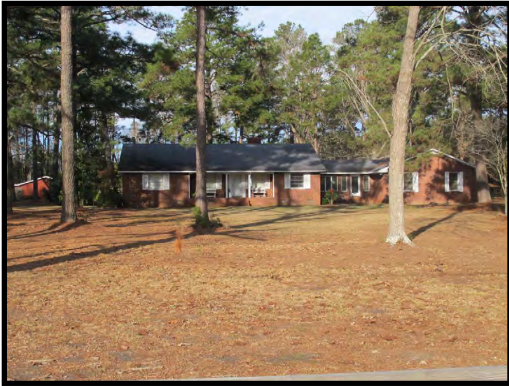
ED1644 – View of House, 3952 Old Battleboro Road, Looking West.
