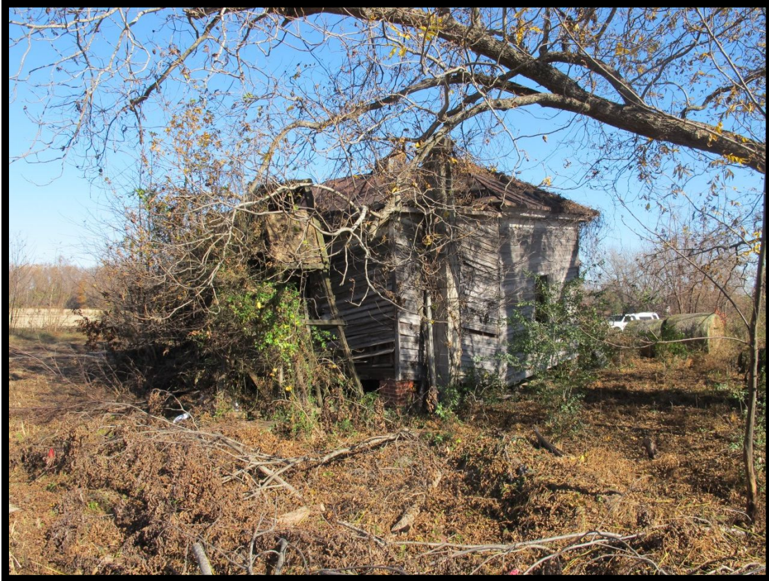
Figure 4.22 Henry Odom Tenant House (F), Looking Northeast
