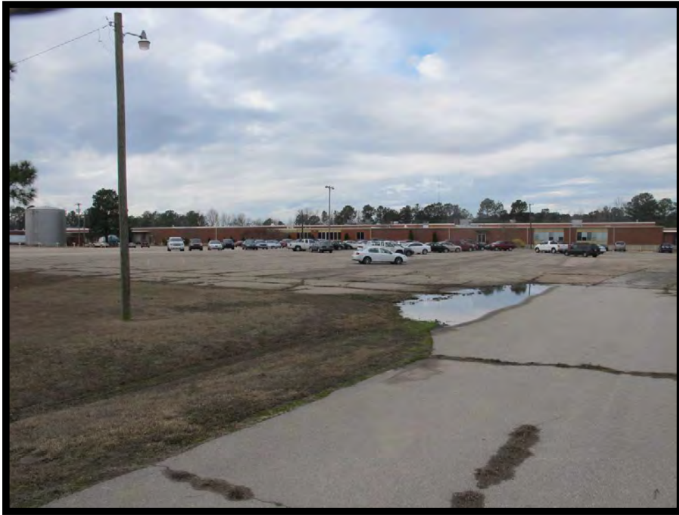
ED1652 – View of Commercial Building, 1450 Atlantic Avenue, Looking Southwest.
