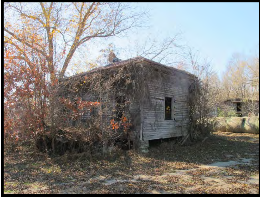
ED0624 – View of Henry Odom Tenant House, Looking Southwest.
