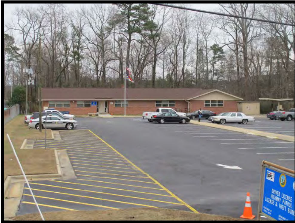
NS1535 – View of Office, 2617 N. Wesleyan Blvd (US 301), Looking Northeast.
