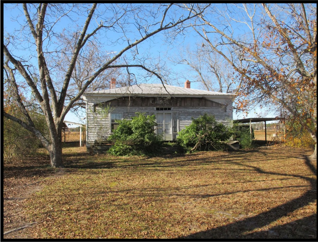
Figure 4.6 Henry E. Odom House (B), Looking West
