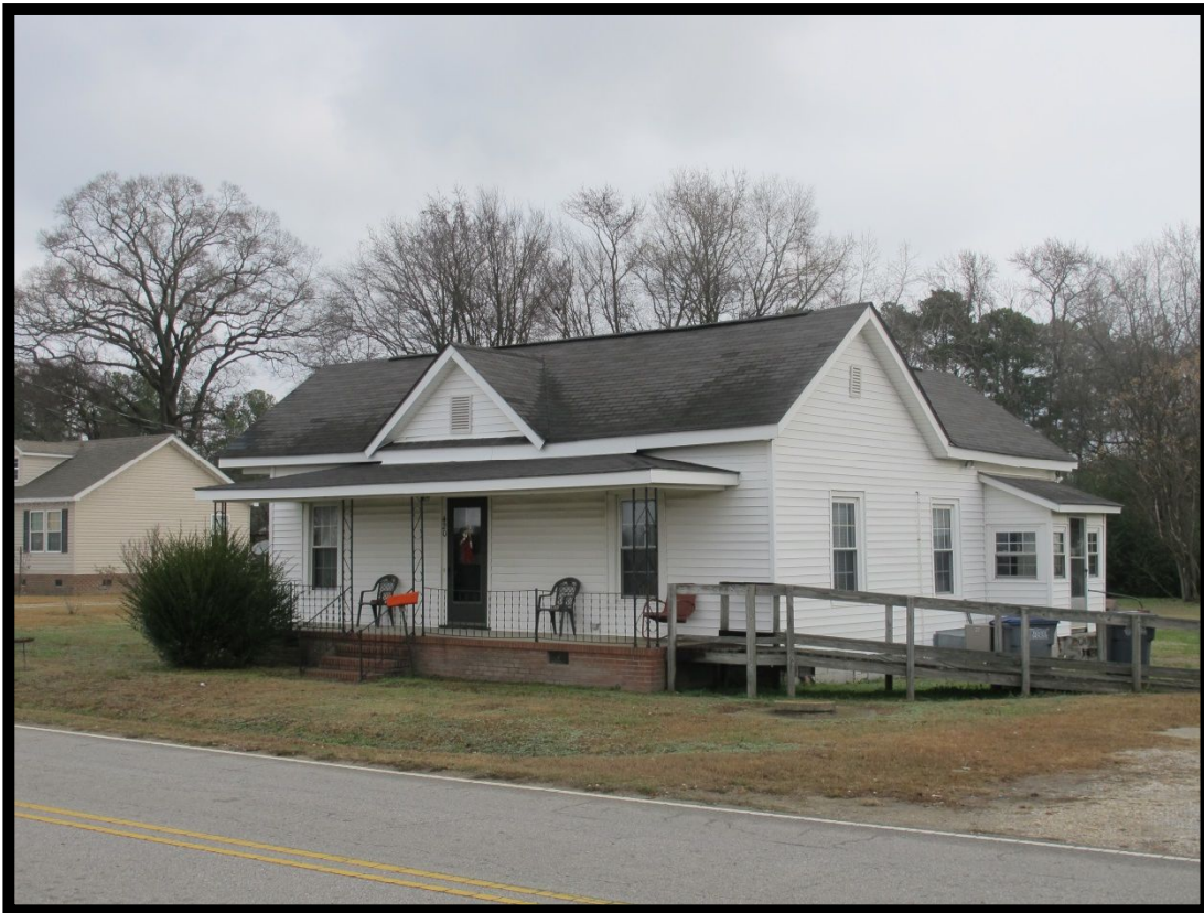
Figure 4.76 House at 420 E Battleboro Avenue (SR 1407), Edgecombe County, Looking North (Not in APE)
