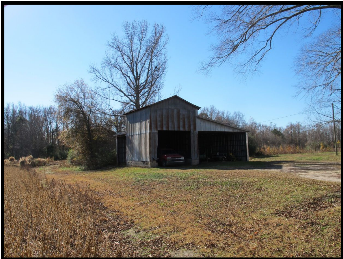
Figure 4.15 Outbuilding (gg), Looking Southwest
