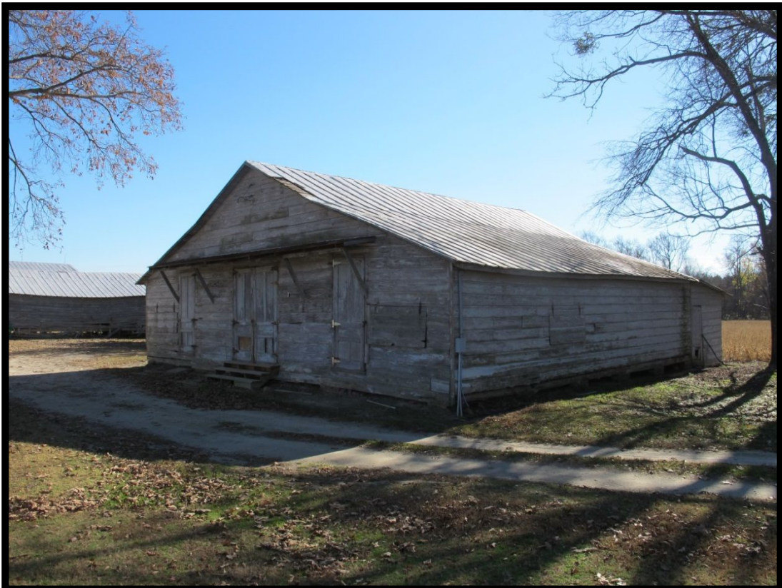
Figure 4.13 Outbuilding (ee), Looking Southeast
